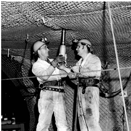
Base CE Miners install rock bolting in UGC. Photo taken by Unknown. Estimated 1967.
